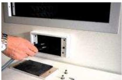
2) Run the cables of the devices which are necessary such as headphones or anything else through the center hole.
