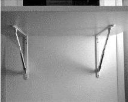
Supported by two folding shelves, it can be easily opened. Just lift it until extending the support mechanism to the limit stop.
